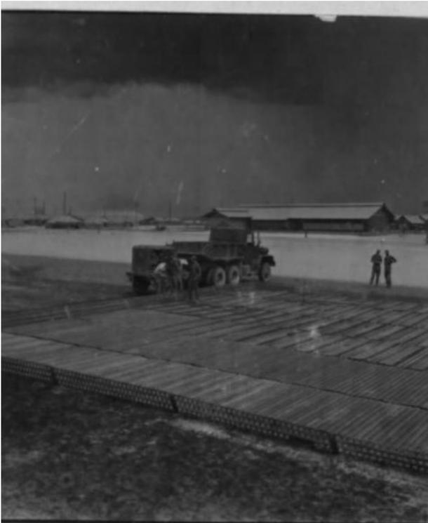
RVN Phu Bai, 1967 a 9 acre Helipad being installed/repared by MCB 121 for the 169th Maintenance Battalion of the 1<sup>st</sup> Cavalry US Army.
